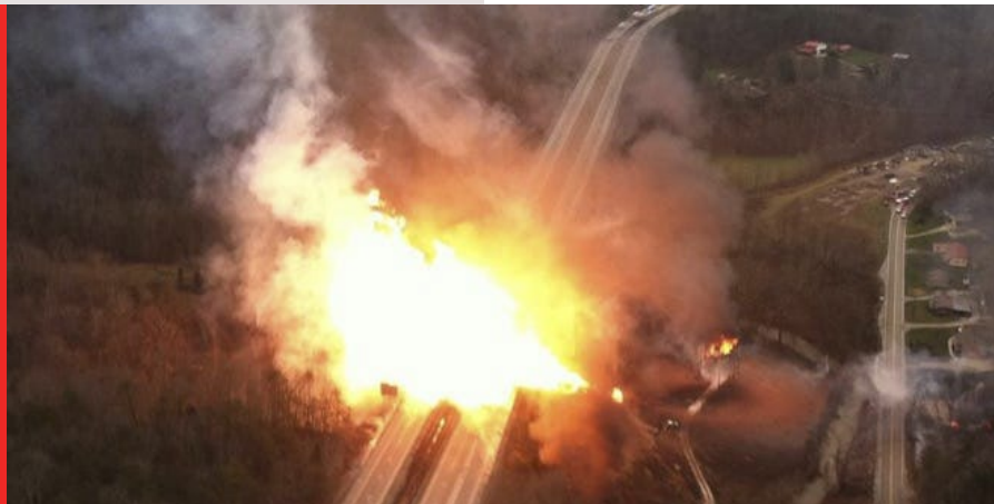
Gas pipeline explosion
